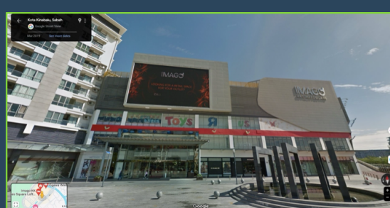
Photo 2: Exterior View of IMAGO Mall
